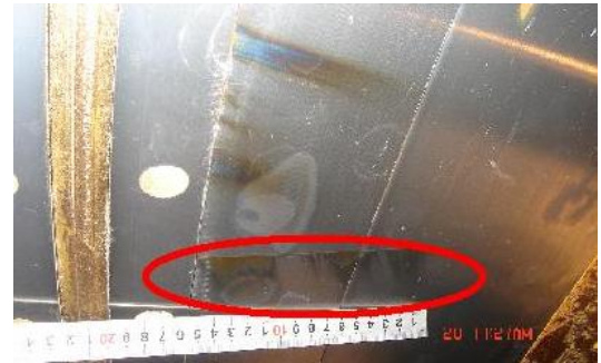
Figure 9 Heated tails observed on the top ring (9F)
